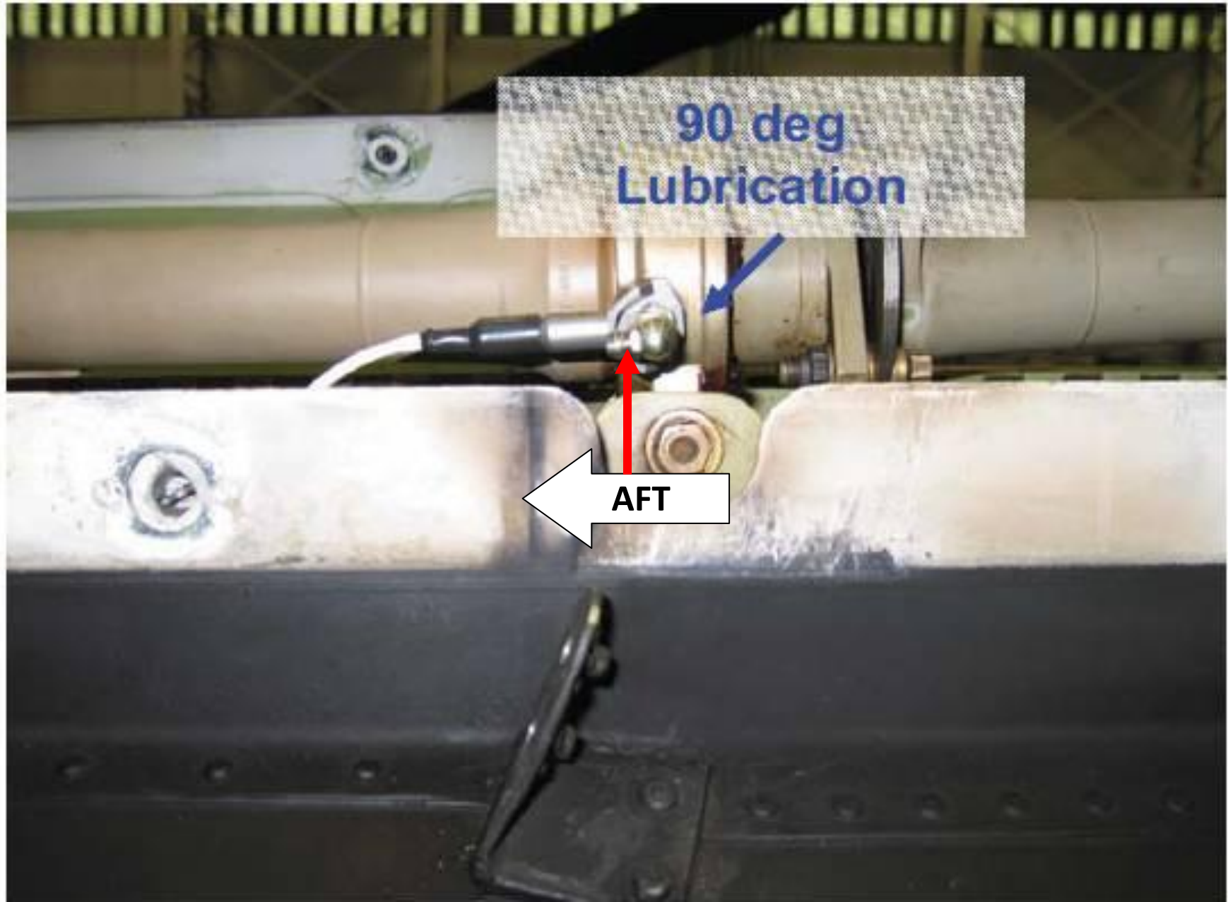
Figure 1: 90 Degree Grease Fitting at Hanger Bearing Number Three (3) Station (STA) 215.05 Installation.
